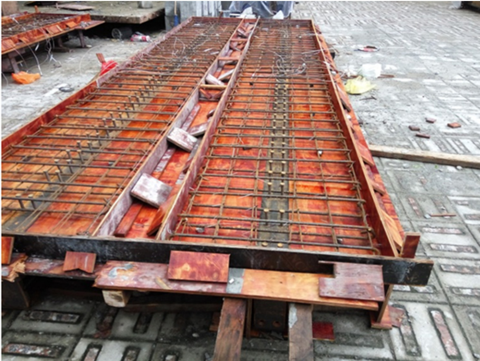
Fig. 2. Illustration of fabricated beam PCB-1 to PCB-4 before pouring of concrete.
